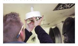
There are no additional brackets or chains. The system that carries the heat and power through the ceiling panels also serves as the mounting system. It even incorporates an adjustable collar, which accommodates different insulated panel thicknesses, from 50mm up to 200mm.
