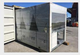
DeltaChill™ - An extremely energy efficient and compact chiller, the DeltaChill™ combines quiet, cost effective scroll compressors and the latest fan technology applied in a modular V-frame coil design.
