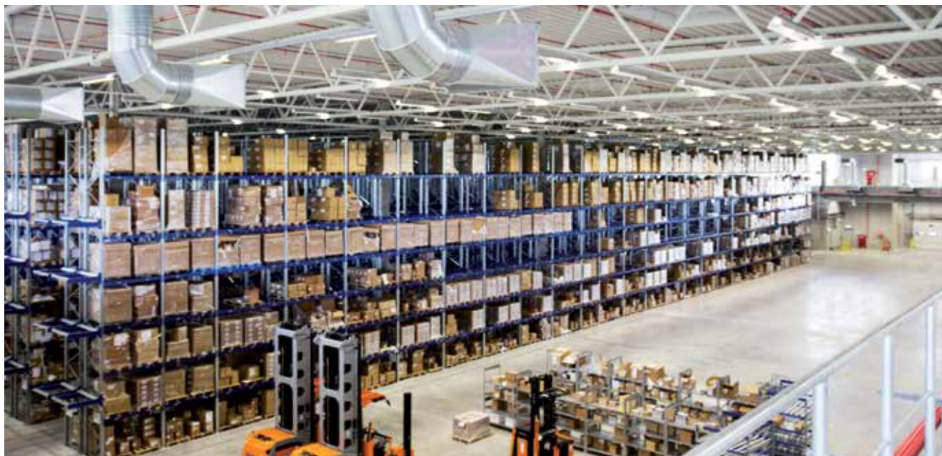
Goods with a value of several million Euros are often stored in high bay warehouses.
